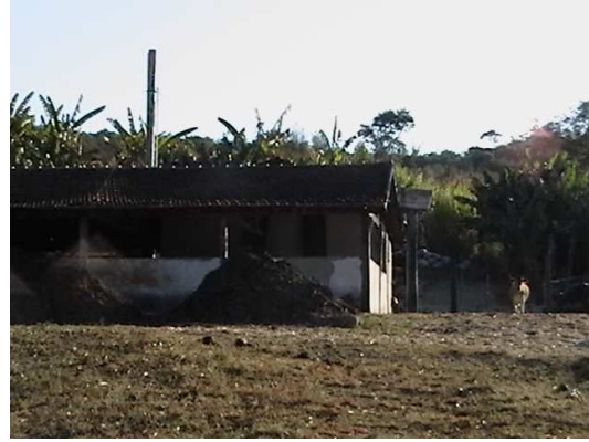
Fig. 2b. Micro-distillery and facilities.
