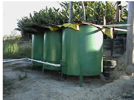
Figure 2f. Batch fermentation tanks.
