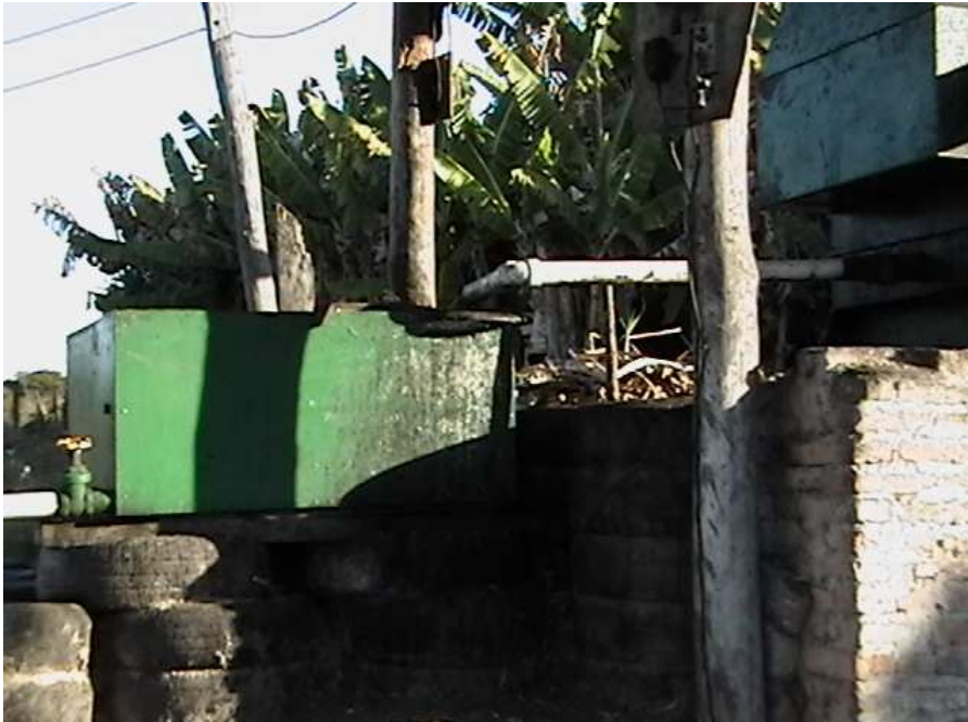
Figure 3e. Dilution tank.
