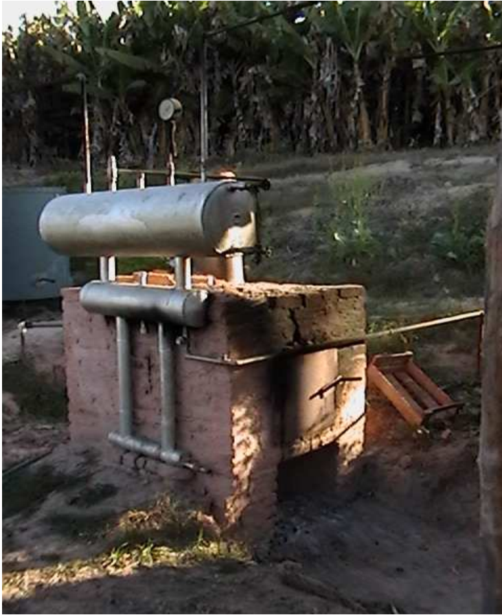
Figure 3g. Firewood furnace.
